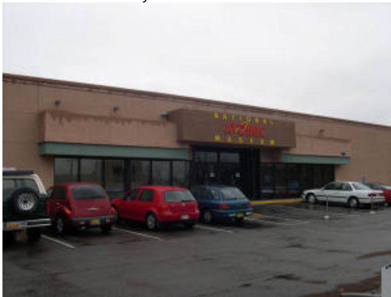
Figure 37. Temporary building of National Atomic Museum. Source: ILE photo.
