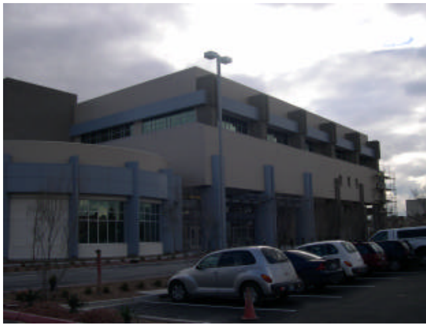
Figure 45. Desert Research Institute Frank H. Rogers Building. Source: ILE photo.
