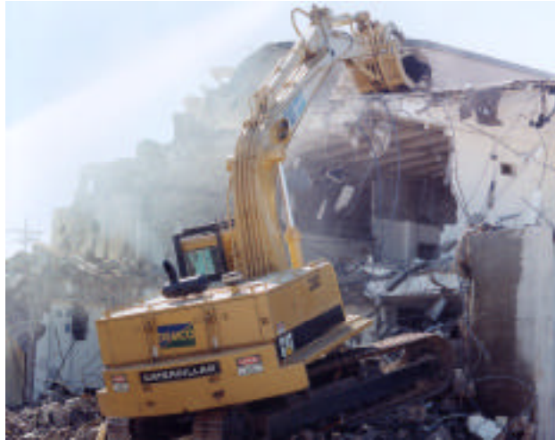
Figure 6. Rocky Flats building being demolished after cleanup. Source: DOE.
