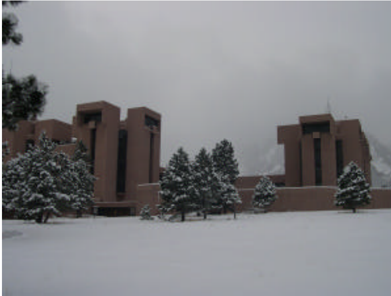
Figure 51. I.M. Pei-designed NCAR building. Source: ILE photo.
